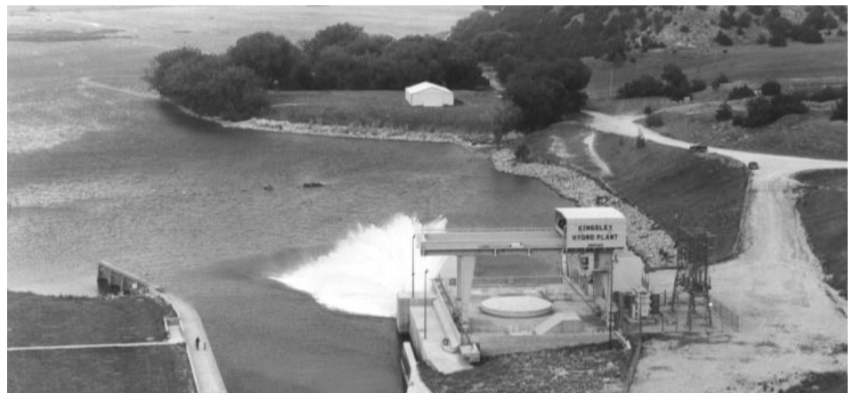
Kingsley Hydroplant — Kingsley Hydroplant, completed in 1984, can generate up to 50 megawatts of electricity. Kingsley and Central's Supply Canal hydroplants — with an additional 63 megawatts of generation capacity — were recently recertified as low-impact hydroelectric power plants.
