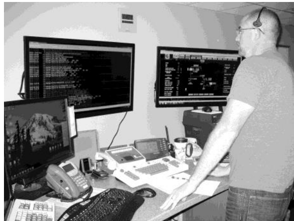
SCADA Upgrade — Assistant Control Operator Logan Ricley controlling water and hydropower operations from the Gothenburg Control Center on the new SCADA system.
